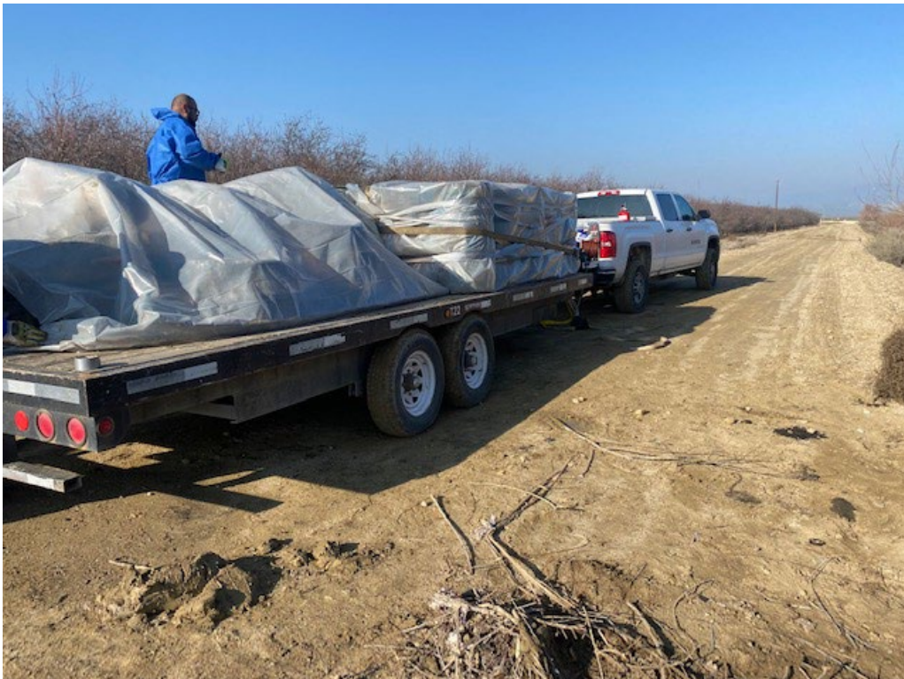
Figure 8. Debris transport and disposal.
